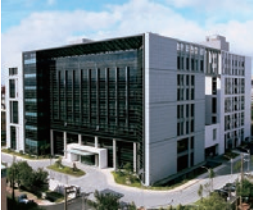
Taoyuan Technology Center (Green Building)
