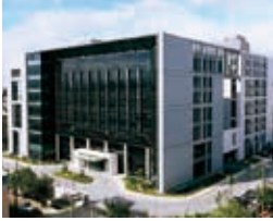
Taoyuan Technology Center (Green Building)
