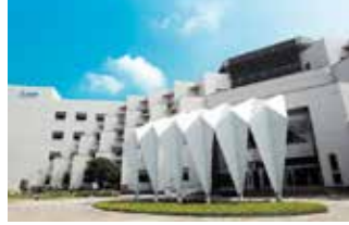
Tainan Plant (Diamond-rated Green Building)
