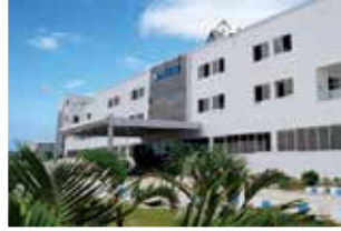
Rudrapur Plant (Green Building)
