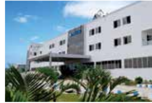
Rudrapur Plant (Green Building)
