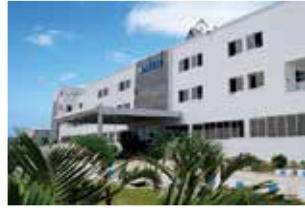
Rudrapur Plant (Green Building)
